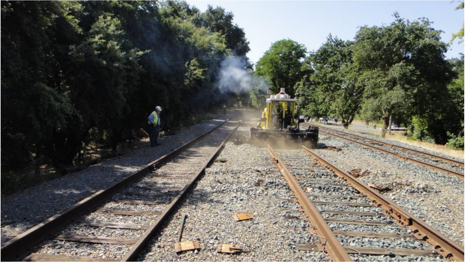
Frank directs Alan in the scarifier following behind the tie-shear to dig out the cribs
