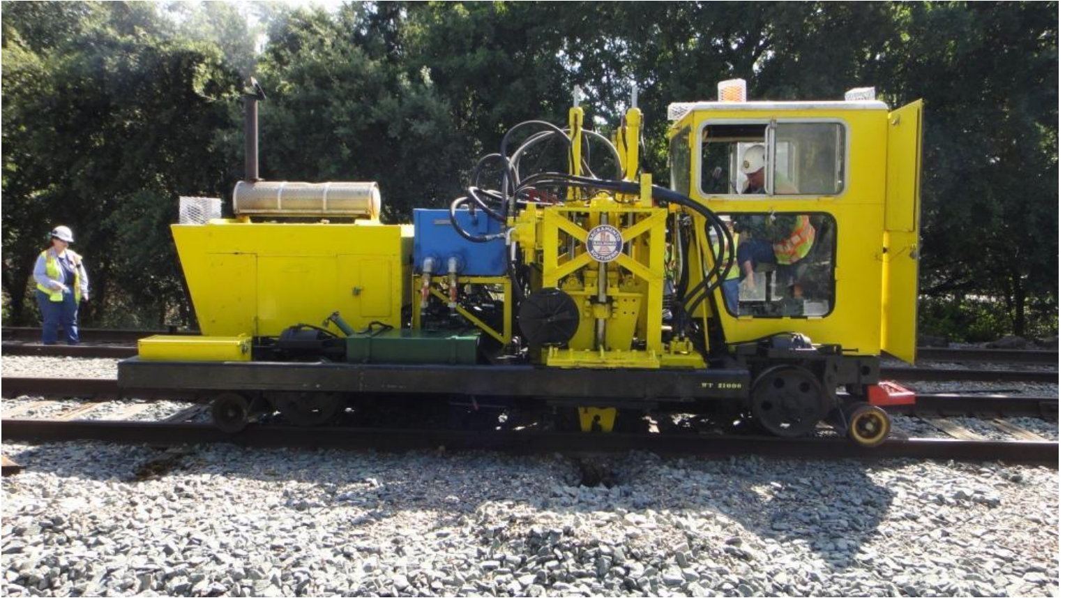
Chris in the tie-shear slices through rotten ties on the Miller Park Siding
