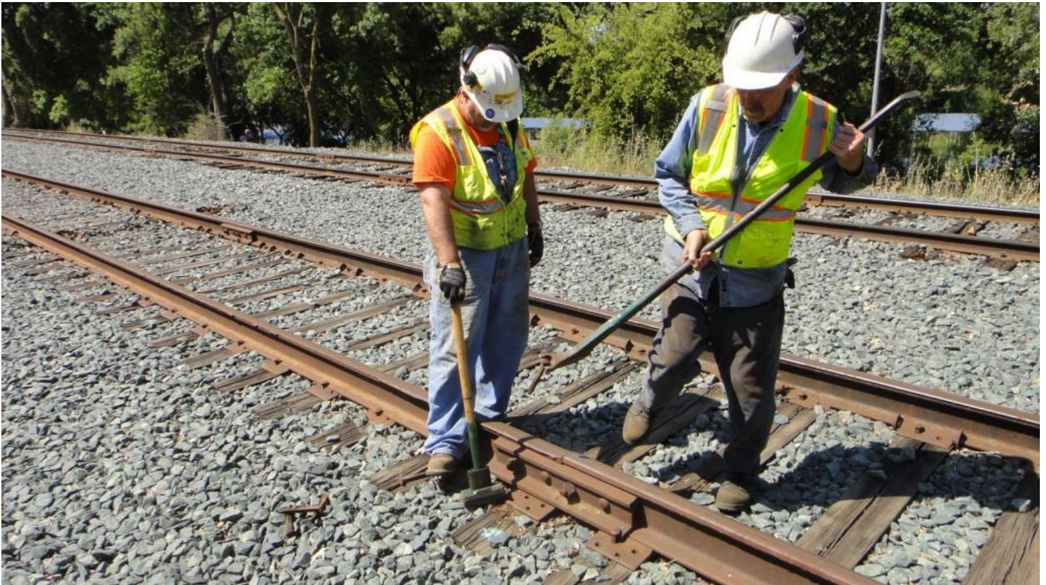
Mike F. and Fred pull spikes and pound out rail-anchors in anticipation of the tie-shear's arrival
