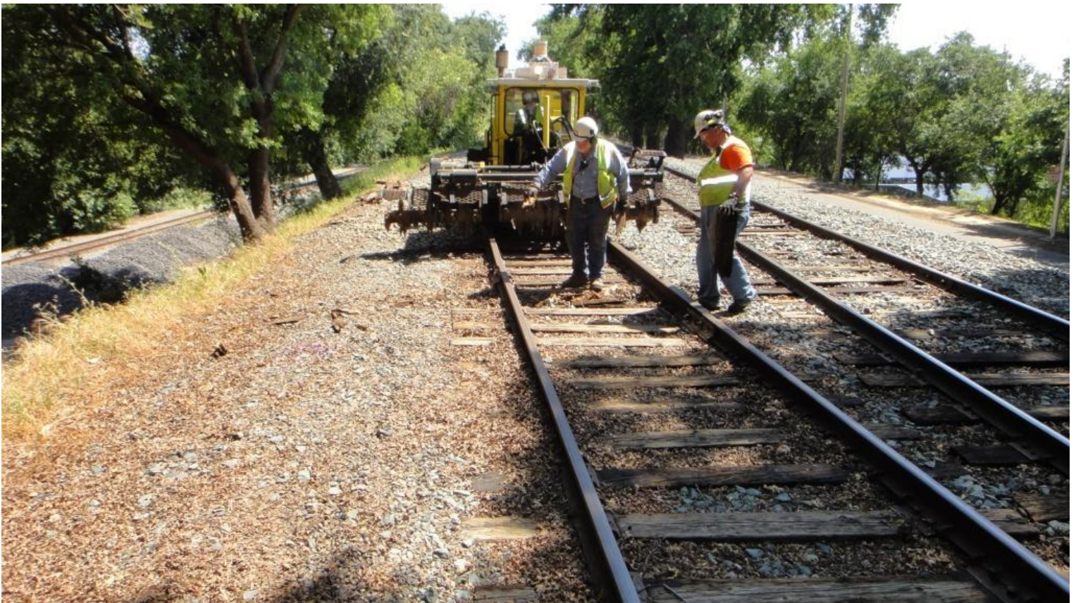
Frank and Mike F. remove tie debris as Alan in the scarifier prepares to come in and dig out the crib
