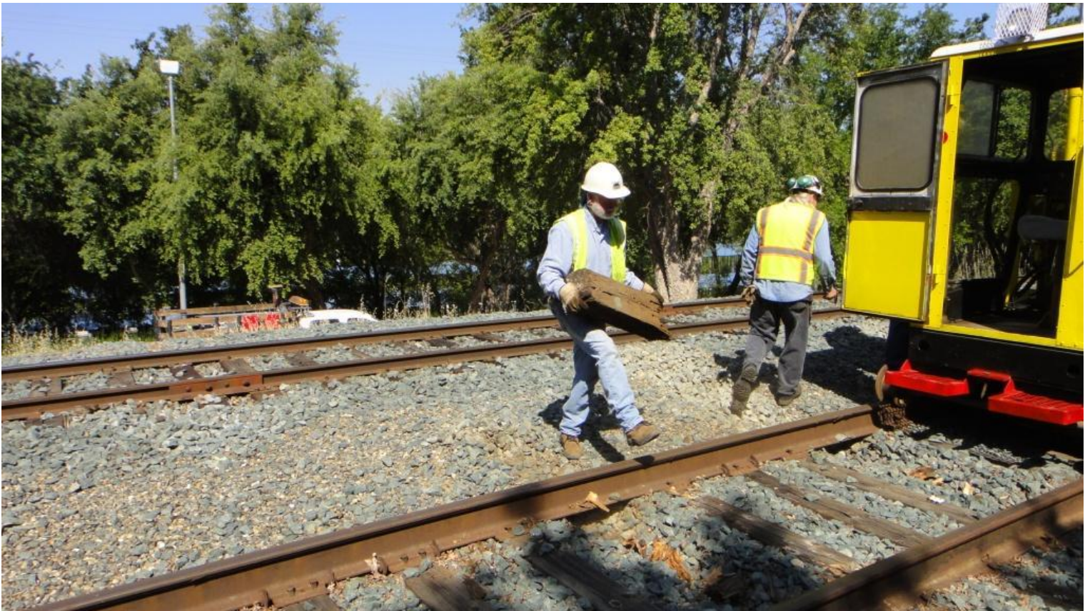
The tie-shear makes tie bits manageable. Mike M. carries off a tie-end after the shear sliced it in three.
