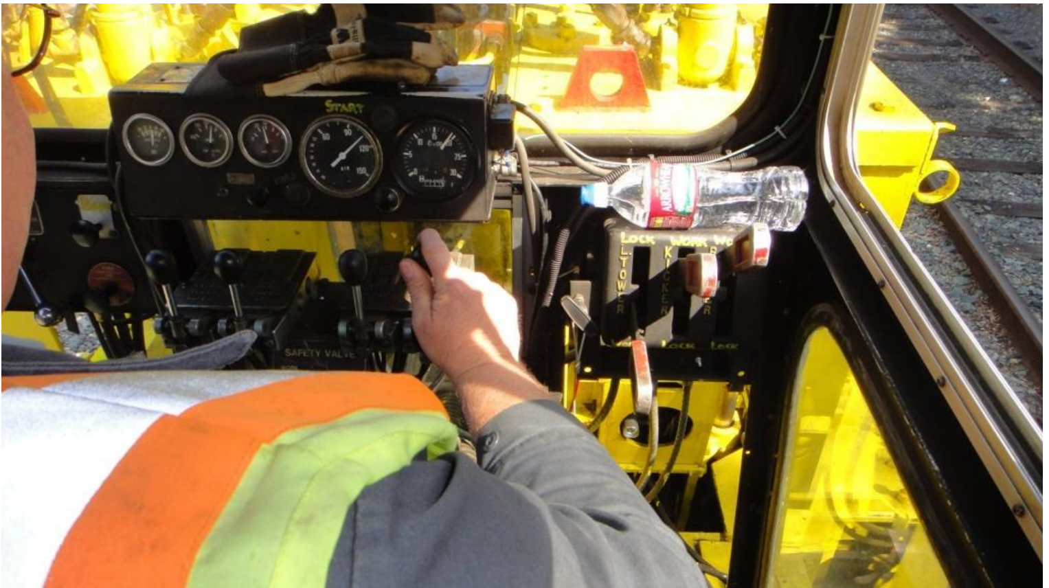
Inside the cab, Chris's nimble touch allows the shear to cut through ties like a hot knife through butter.
