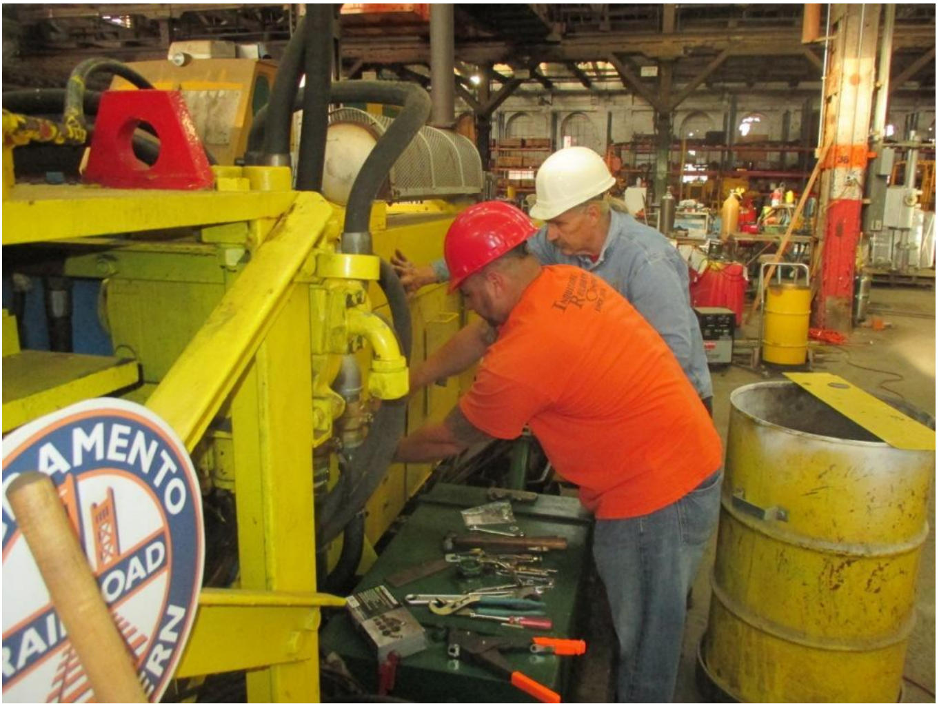
Joe and Fred install the shroud on the tie-shear
